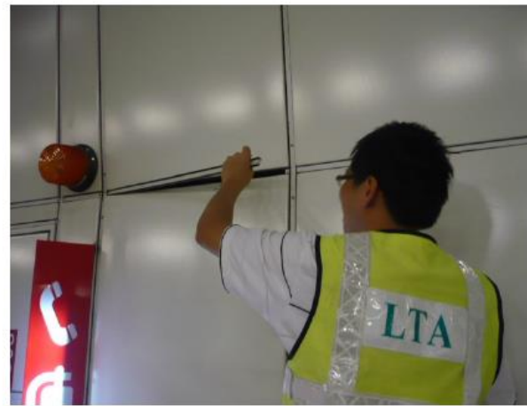
2. Pull out the tension plate for lower cladding
