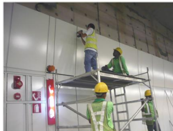
4. Unscrew and remove the tension plate for the top cladding
