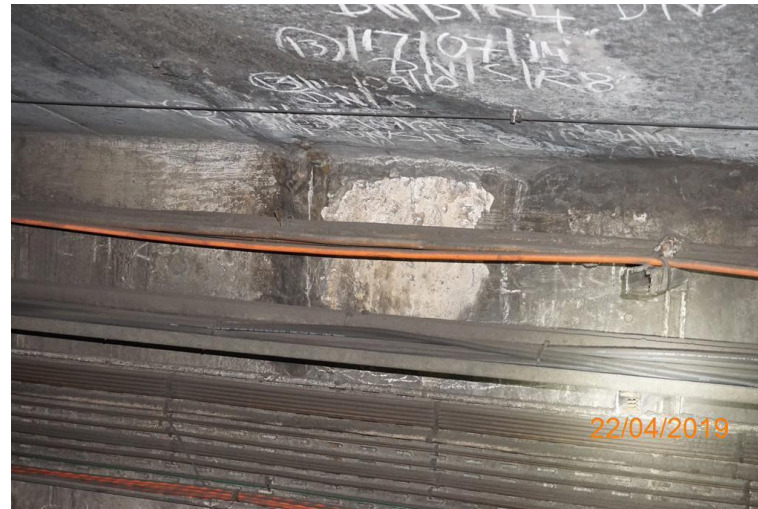
Concrete spalling
