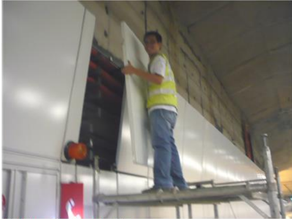
5. Lift up the top cladding
