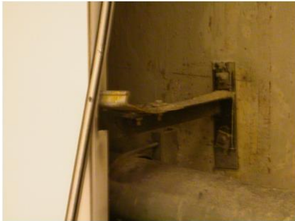
Showing the brackets to hold the cladding. Width approx. 300mm
