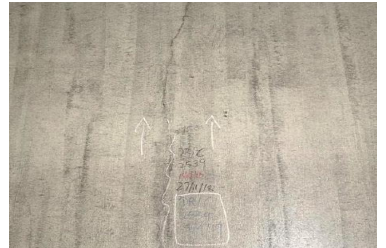
Surface cracks
