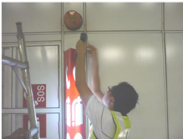
1. Take out the screw on the tension plate lower cladding
