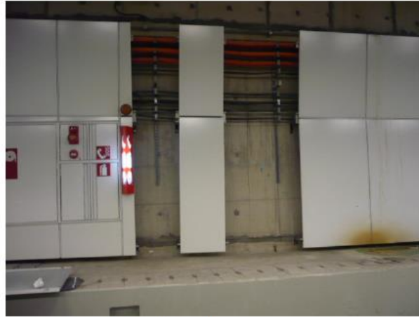
6. Cladding after taking off
